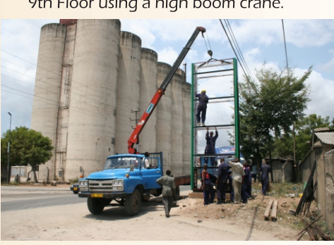
160 sq Feet Flexy Sign being installed on the 9th Floor using a high crane.
